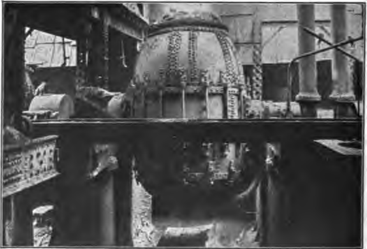
FIG. 114.—Bessemer converter, in action.
